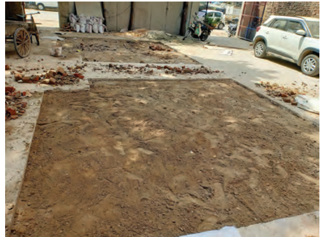
Concrete pathway work in progress in front of the Chowki building
