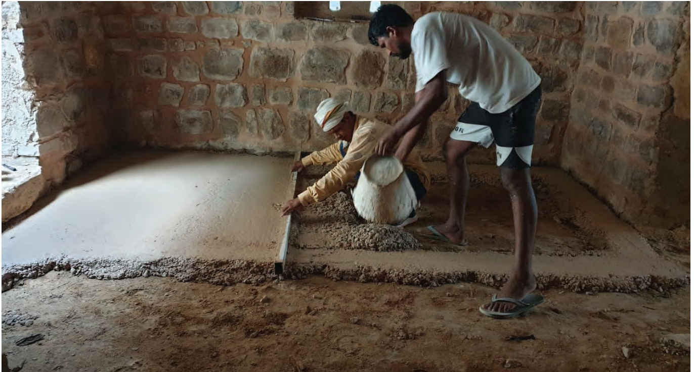
Flooring in progress in the chowki
