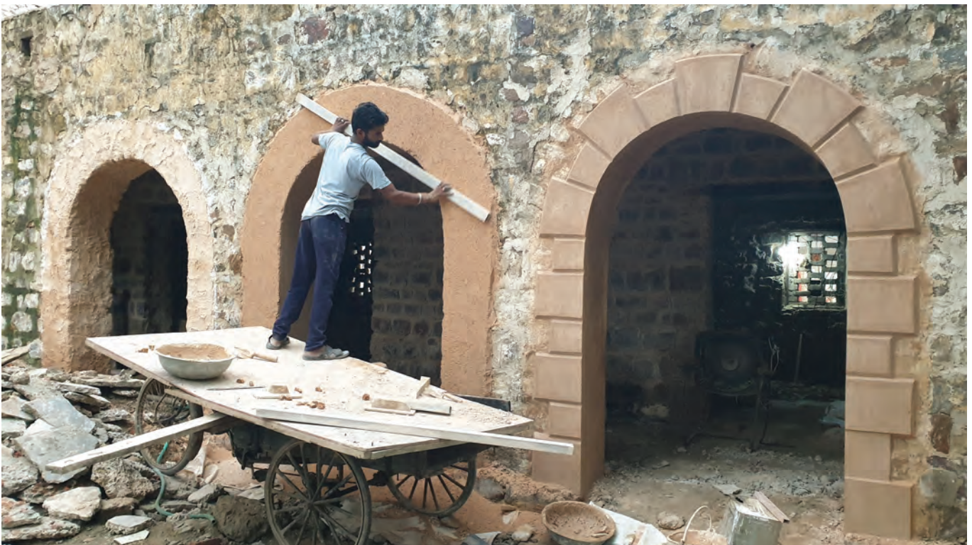
Barh ki Chowki Site during Phase-II works
