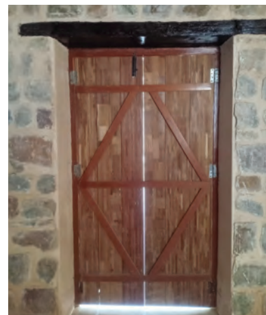
Making and installation of Teak wood doors
