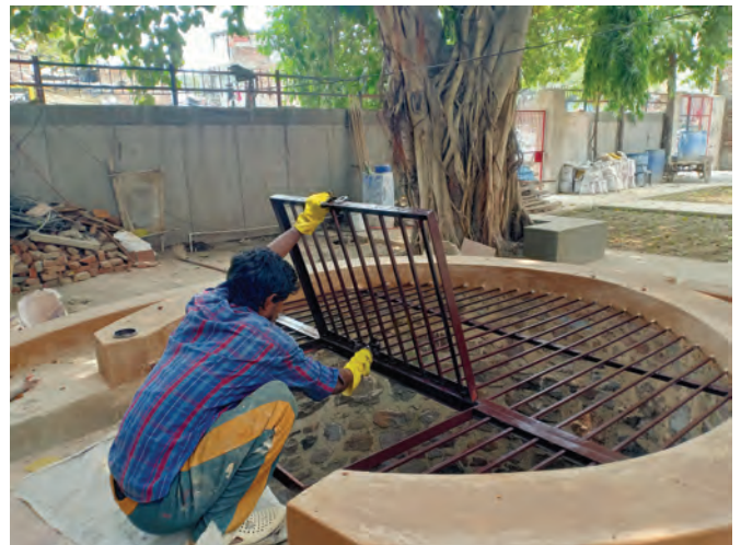
Well during installation of metal cage
