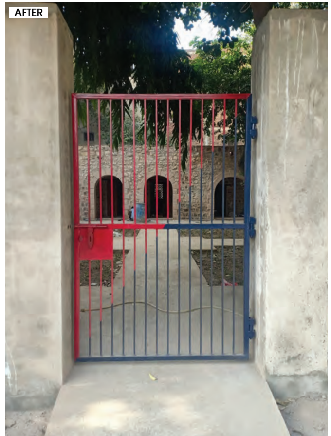
Barh ki Chowki entrance gate
