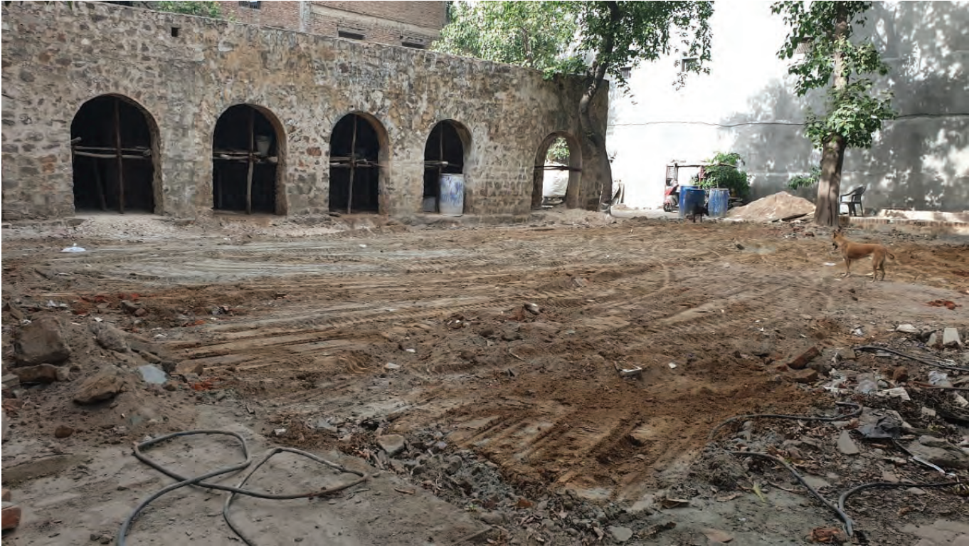
Barh ki Chowki Site during Phase-II landscape works
