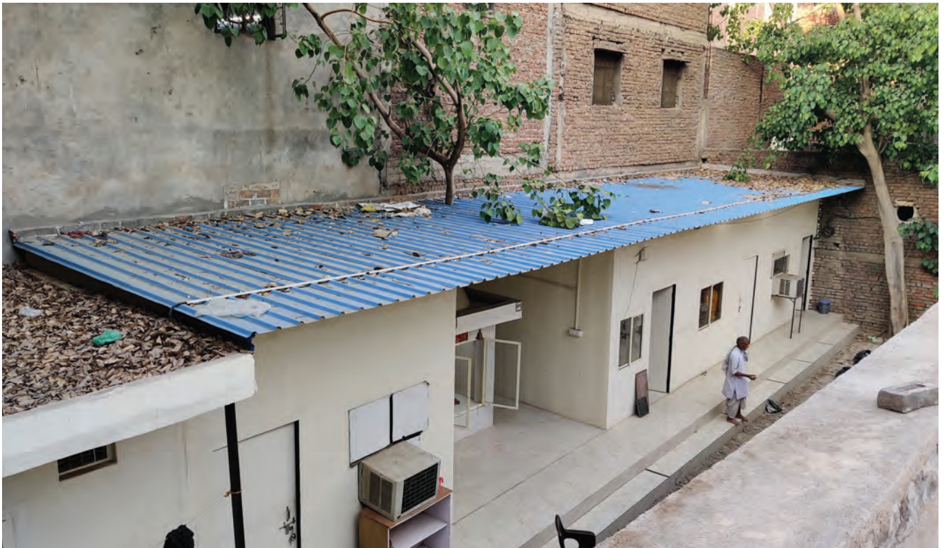
Porta Cabins constructed behind the Chowki building
