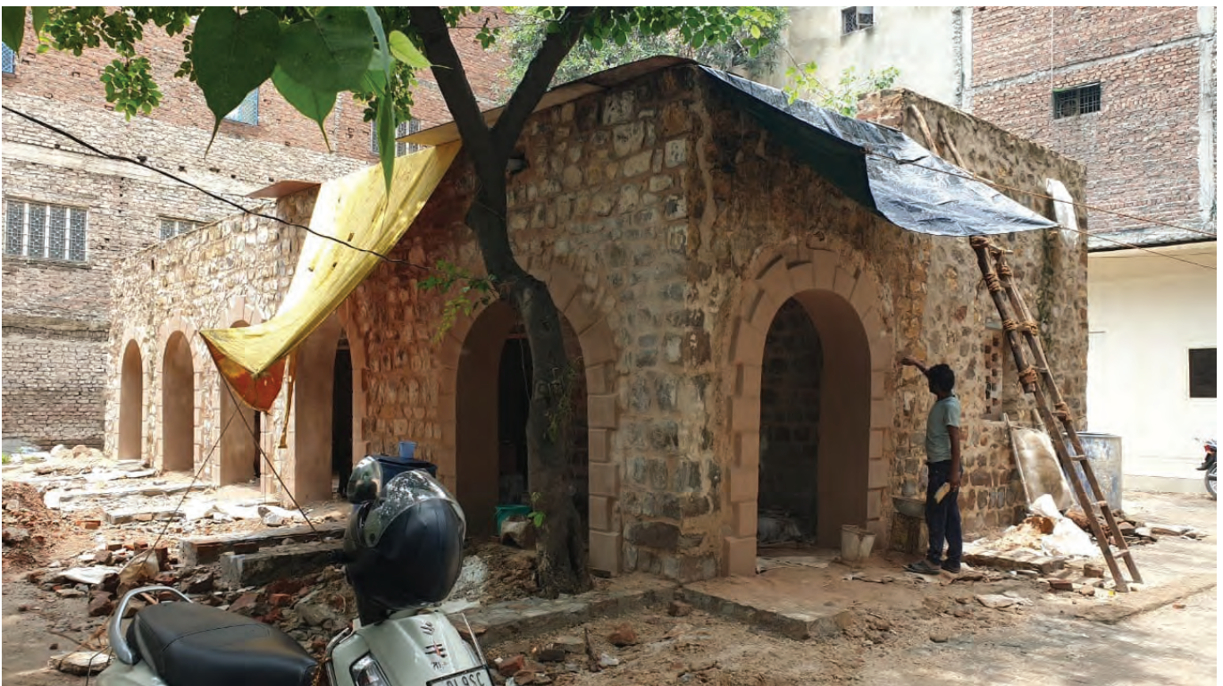
Barh ki Chowki Site during Phase-II works
