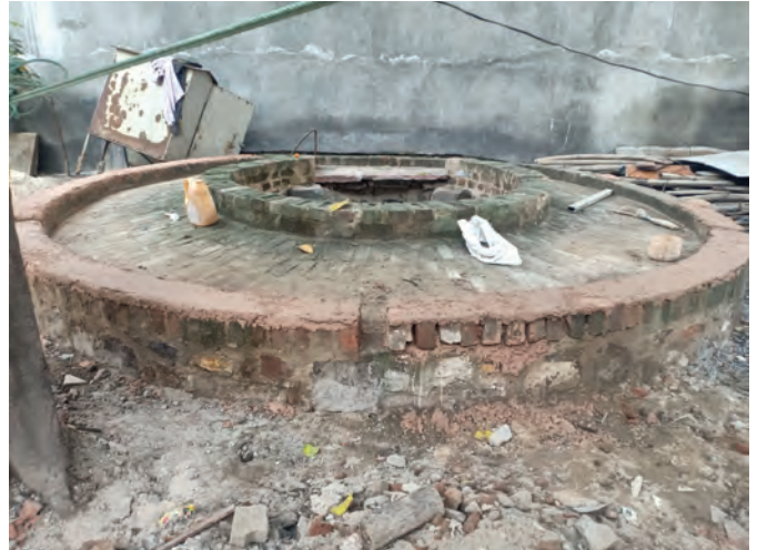
Well during restoration
