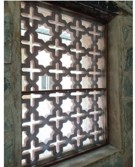
Installation of Red Sandstone window jali and mosquito mesh
