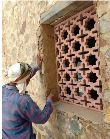
Installation of Red Sandstone window jali and mosquito mesh
