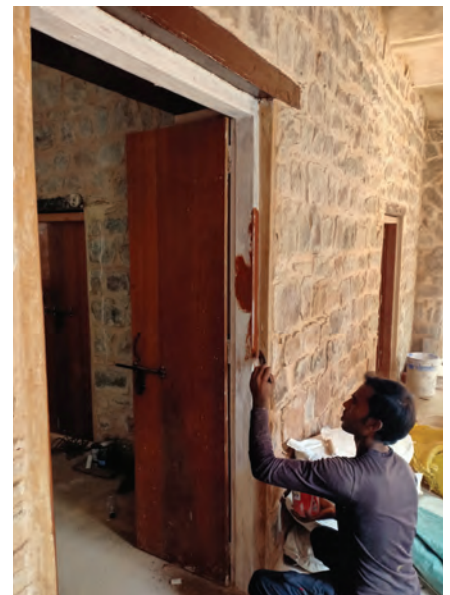
Making and installation of Teak wood doors
