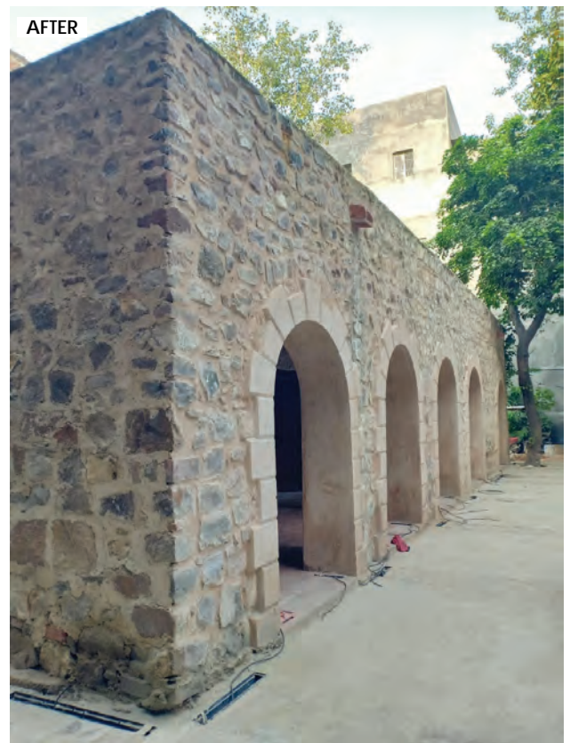
Barh ki Chowki external facade
