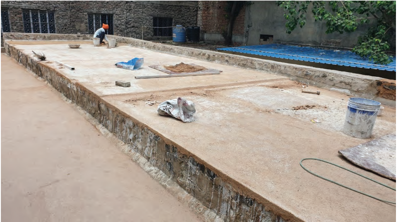
The application of lime mortar on the roof
