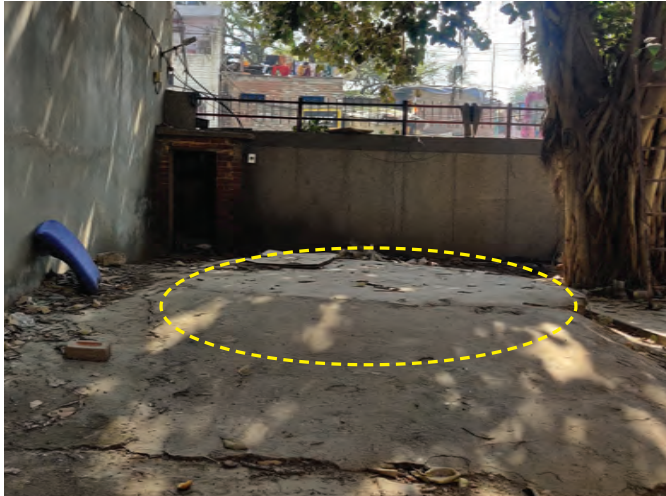
Well before opening up the slab
