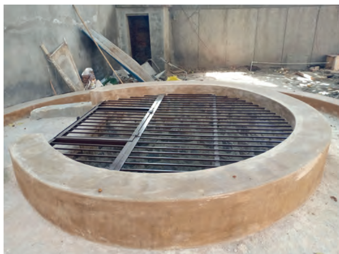
Well during installation of metal cage
