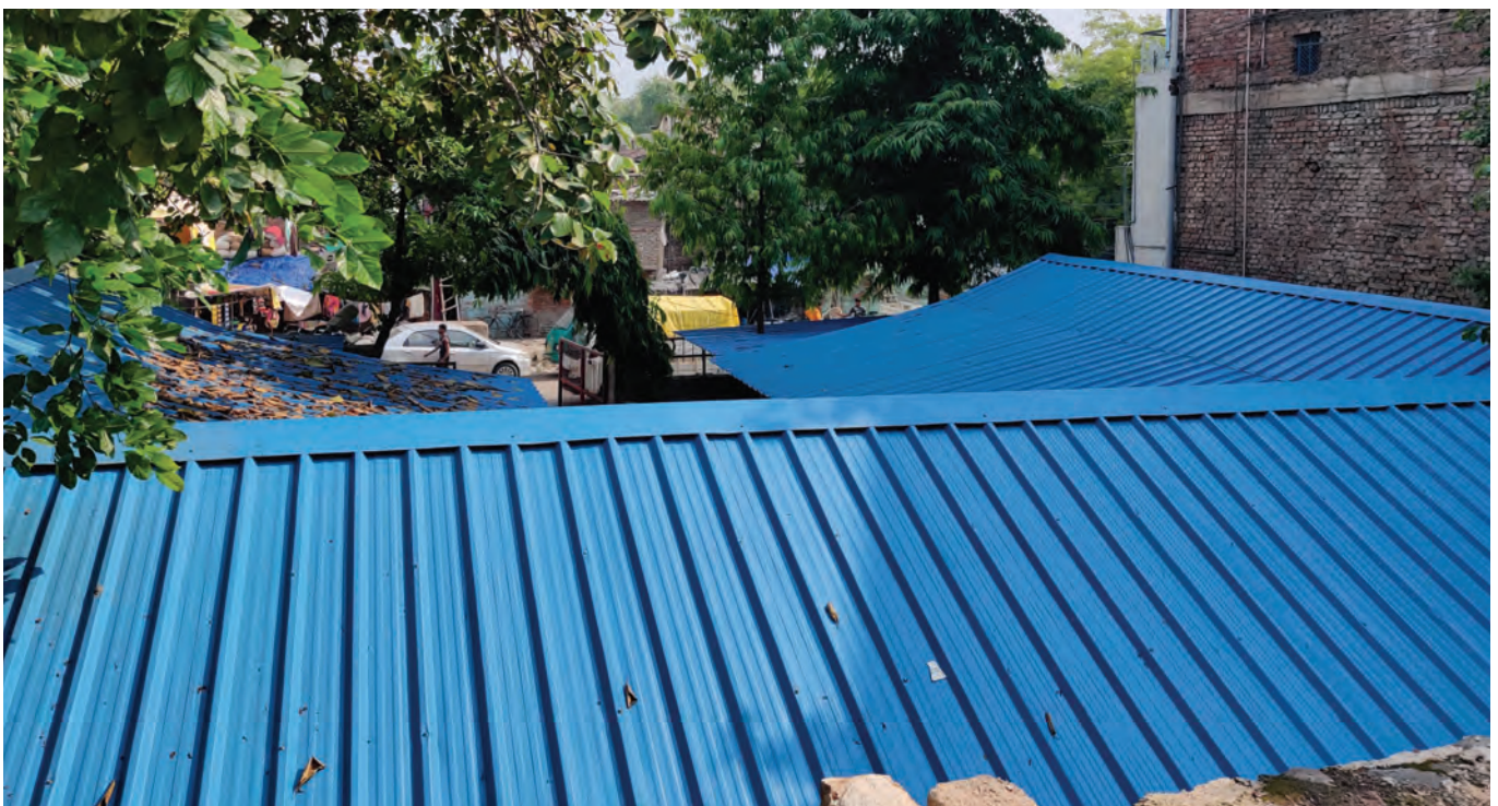
Existing Porta Cabins in front of the Chowki building
