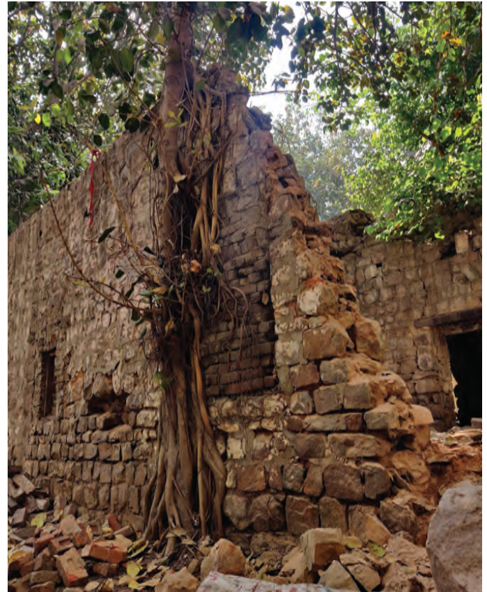
View of Barh ki Chowki front facade, February 2023
