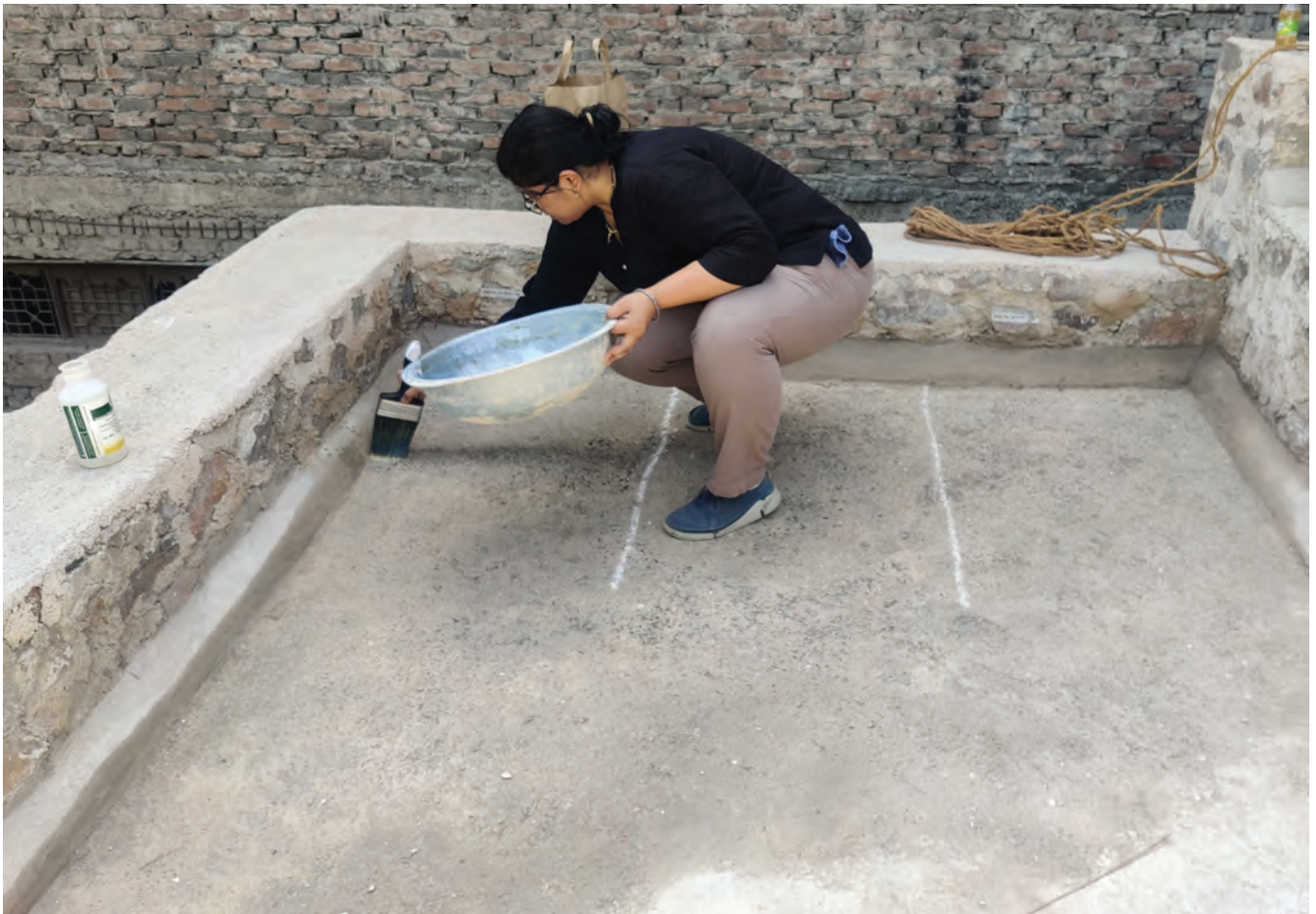
Testing of waterproofing samples for the roof
