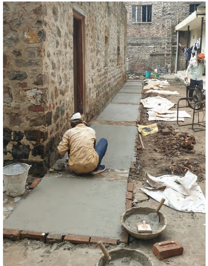
Plinth protection around the periphery of the structure
