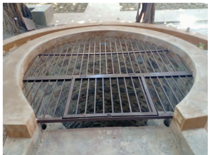
Well post restoration
