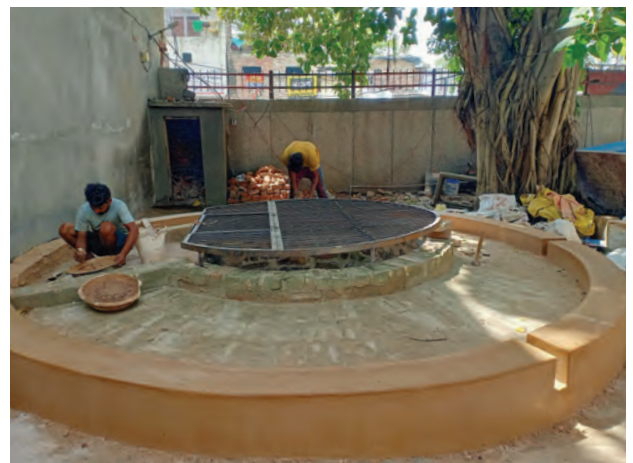
Metal cage addition and plaster of the well
