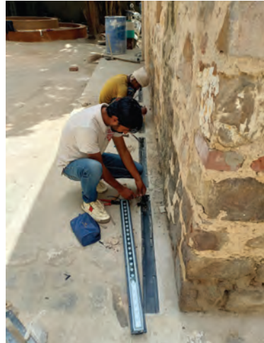
Installation of the lighting fixtures on site
