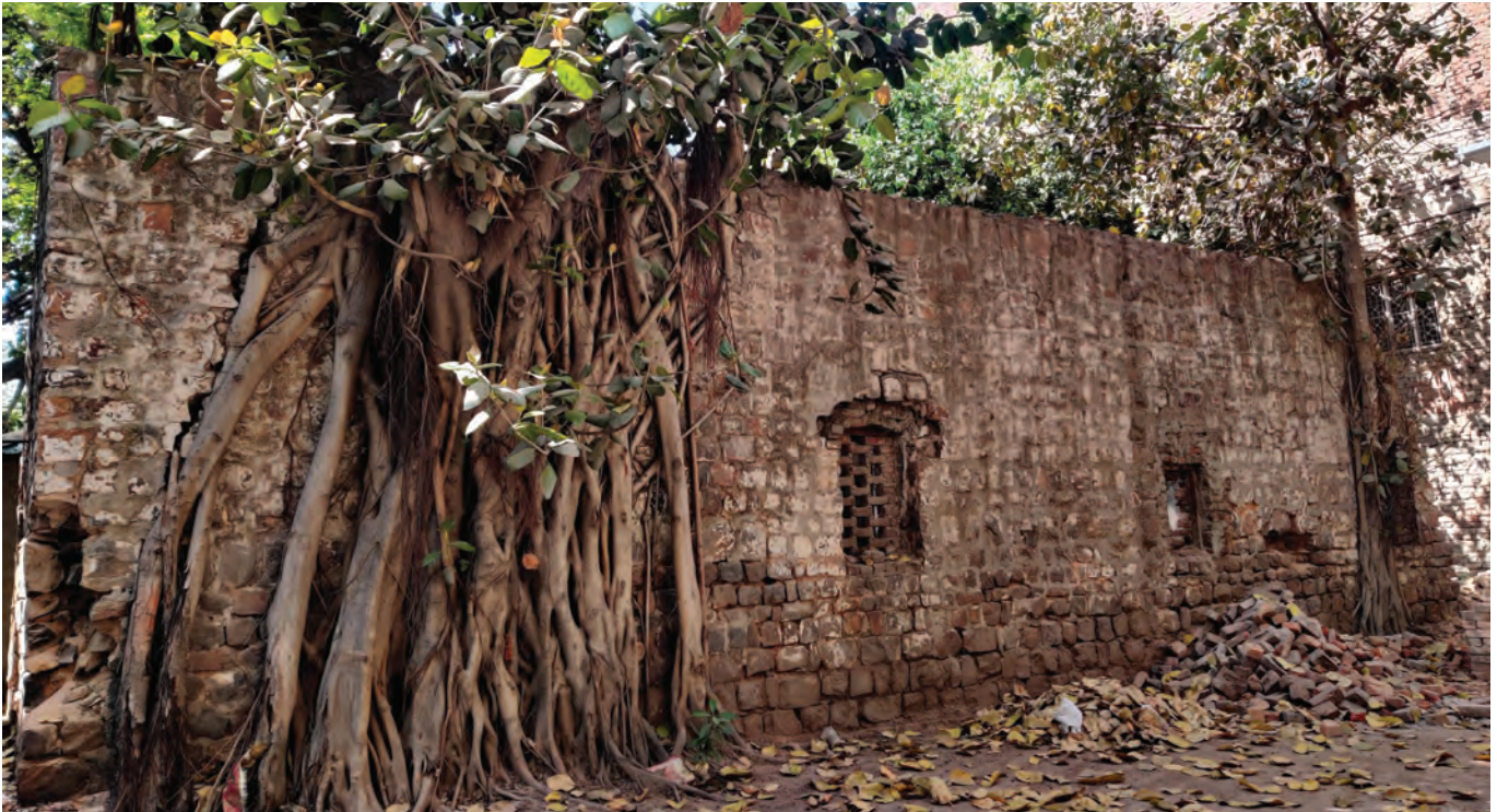
Barh ki Chowki before restoration, April 2022
