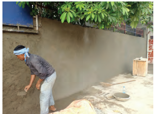
Cement repairs of the compound wall
