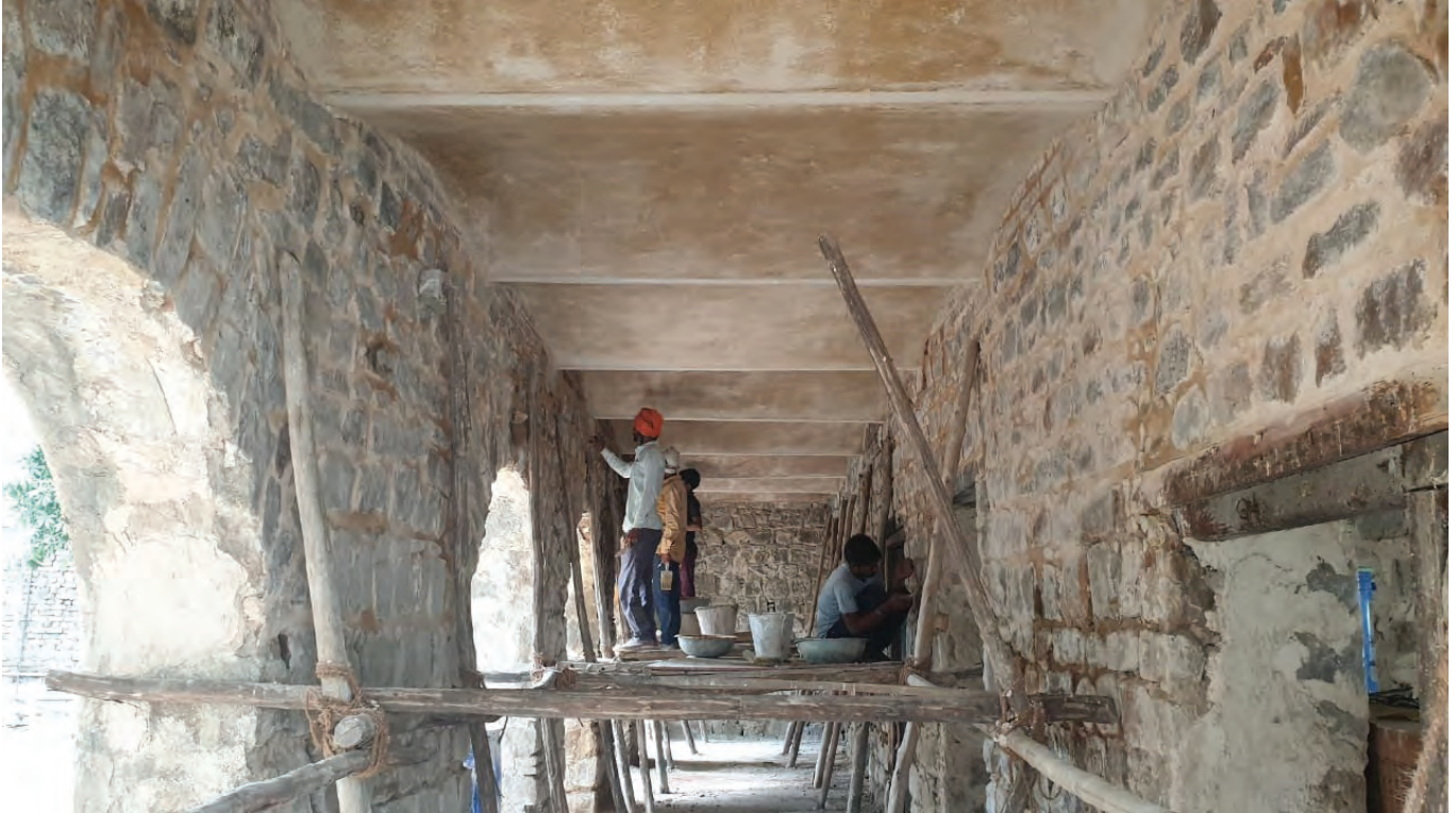
Barh ki Chowki Site during Phase-II works
