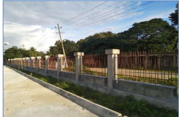
Boundary Wall, Bengaluru, Karnataka
